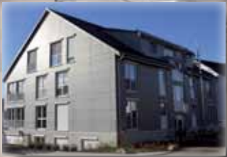
Gelungene Symbiose aus moderner CNC-Technik & Zimmermannstradition Modern CNC technology and traditional carpentry in perfect harmony
